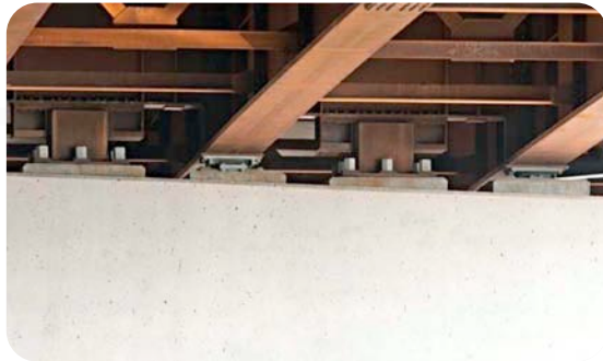
Pot bearings with fuses to free movement during an earthquake
